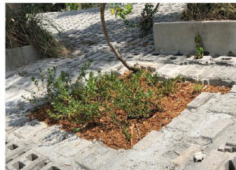
City of Sarasota Indian Beach Revetment Wall Repair and planting
