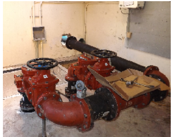
View inside Lift Station 21
