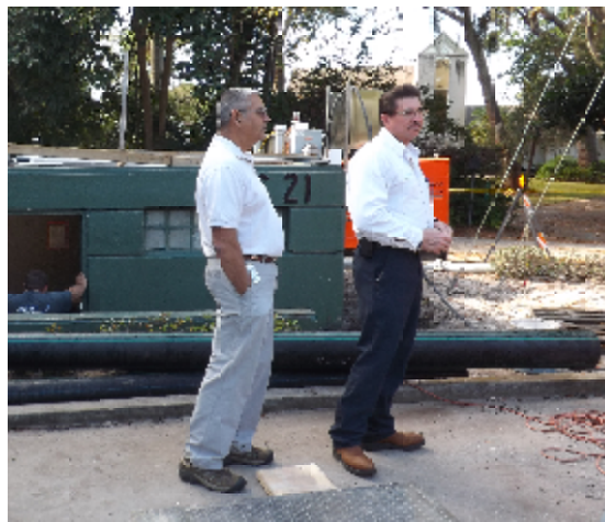
John Chapman, right, checks Lift Station progress.
